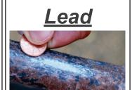
If the pipe is silvery gray and, 1) is easily scratched, 2) the metal seems soft, and 3) a magnet doesn't stick to it, you likely have a lead pipe.
