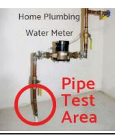
Your water meter could be located inside your home's basement or crawlspace. The service line will enter the house from underground through the floor or foundation wall, before connecting to the water meter. There will be shutoff valves on one or both sides of the water meter. Residential service lines are <sup>3</sup>/<sub>4</sub> to 2 inches in diameter.
